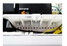
1. Determine where shelf is to be installed and secure to back wall of FMC using provided screws.
