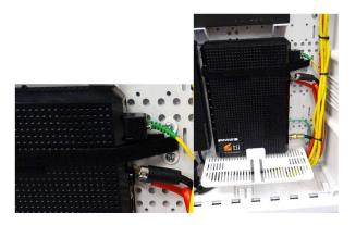
Secure component to back wall using Velcro<sup>™</sup> and clips.
